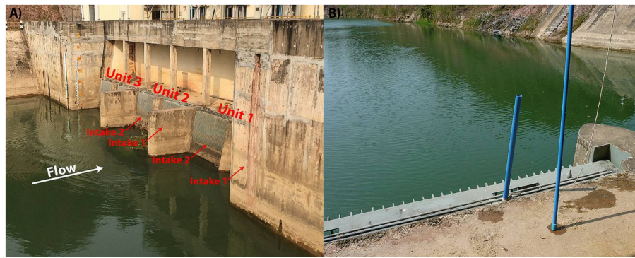
Figure 3. Nam Song Dam forebay showing: (A) turbine unit numbering; (B) Polyvinyl chloride (PVC) release pipe and plunger.
